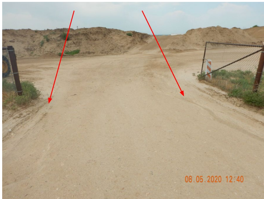
Photo 3. Photo taken from the main point of access to the facility, facing West. Photo illustrates unmanaged stormwater run-on onto the facility. Note: There was stormwater run-off from the southern facility.
