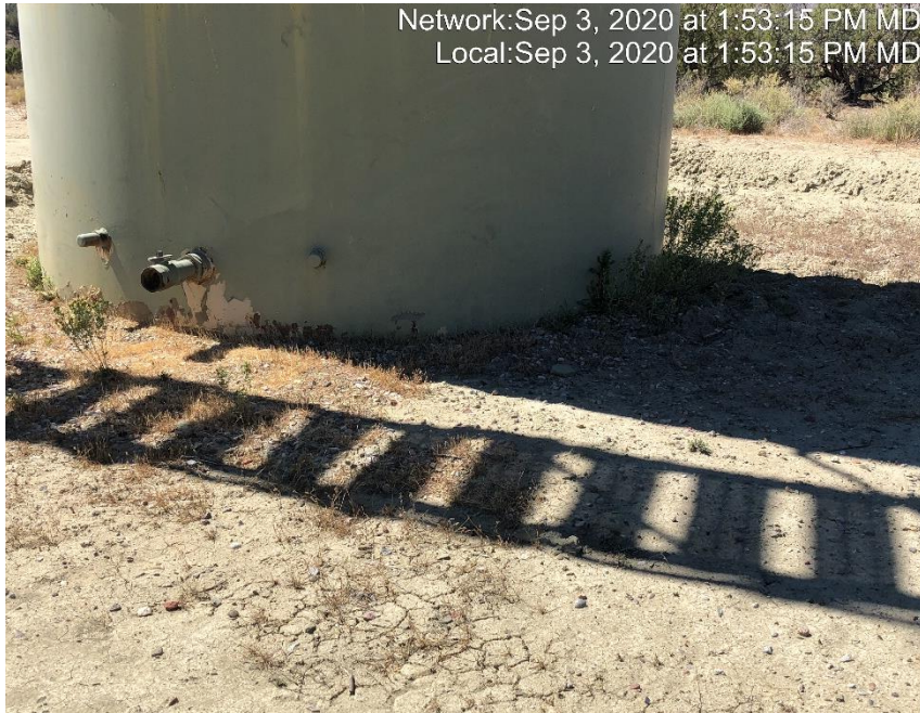
Photo #1846 Weeds growing inside tank containment.
