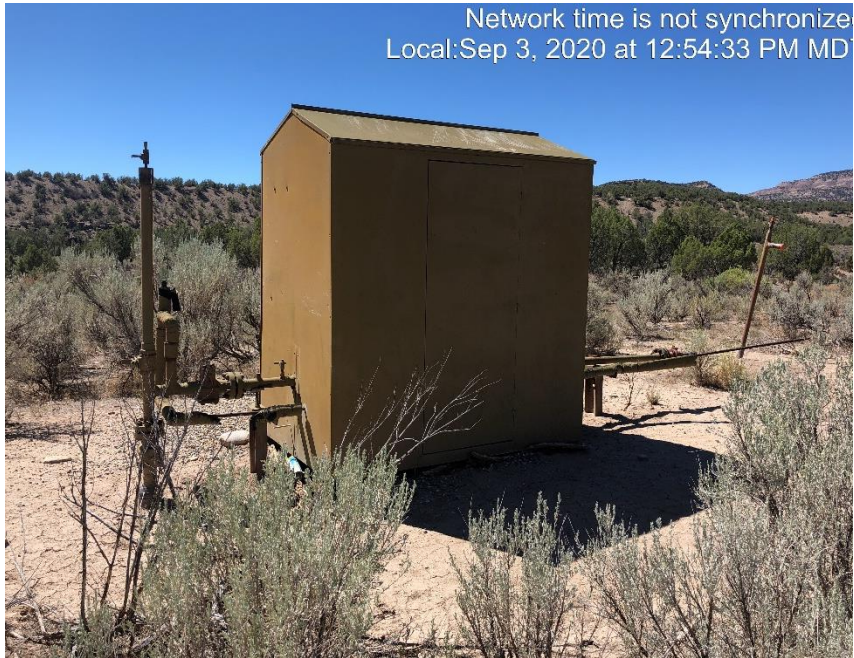
Photo #1844 Unused meter run.
