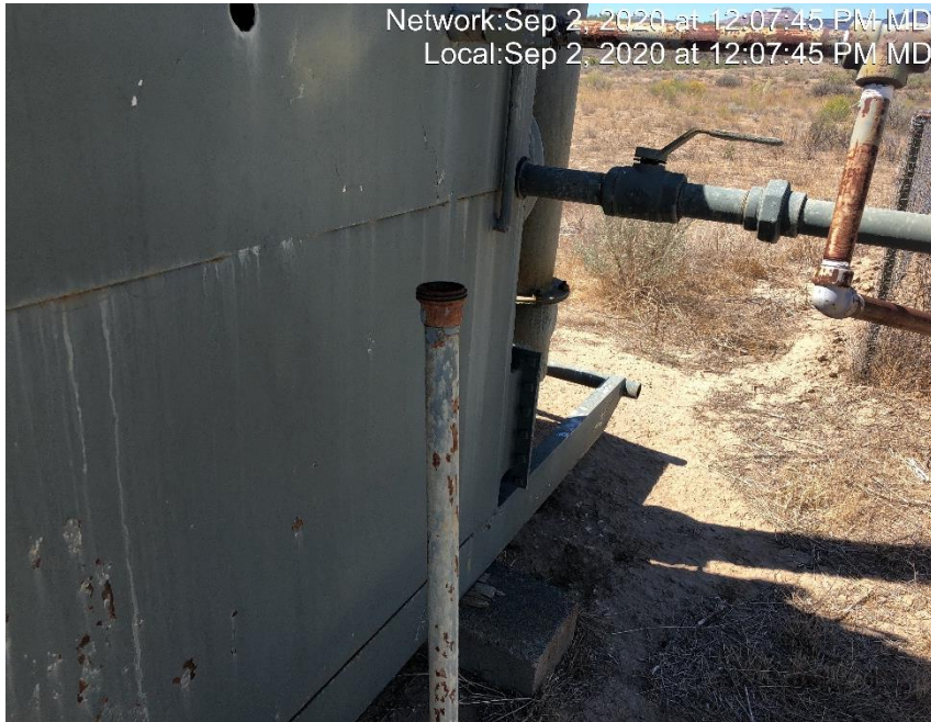
Photo #1832 Flow line risers not LO/TO.
