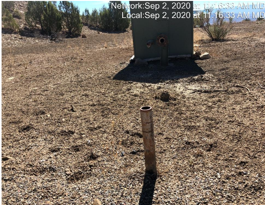
Photo #1828 Flow line riser not LO/TO.
