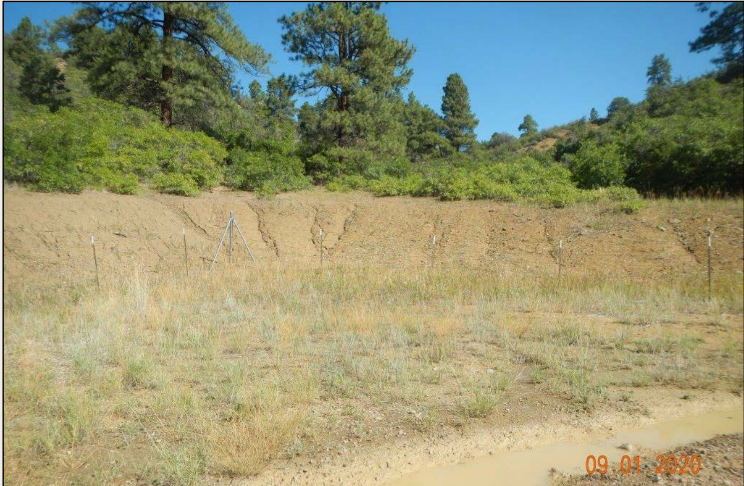
Photo 3. View of the northwestern project area. Bare soils need stabilization.
