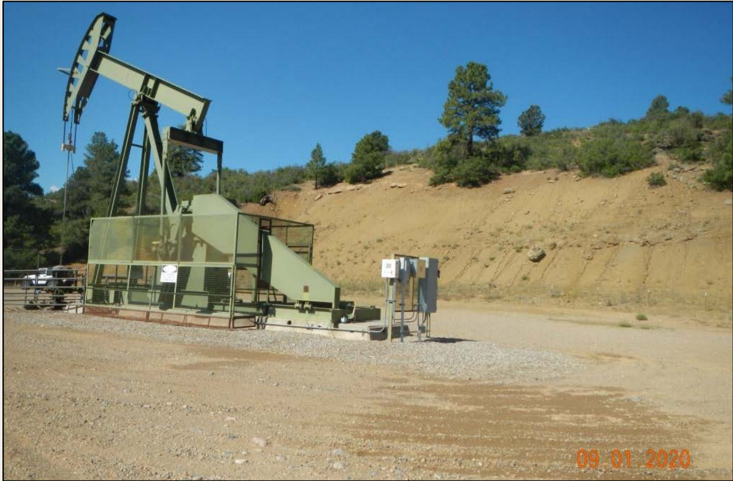
Photo 4. View of the well pad cut-slope. Additional stabilization measures are needed to stabilize bare soils.
