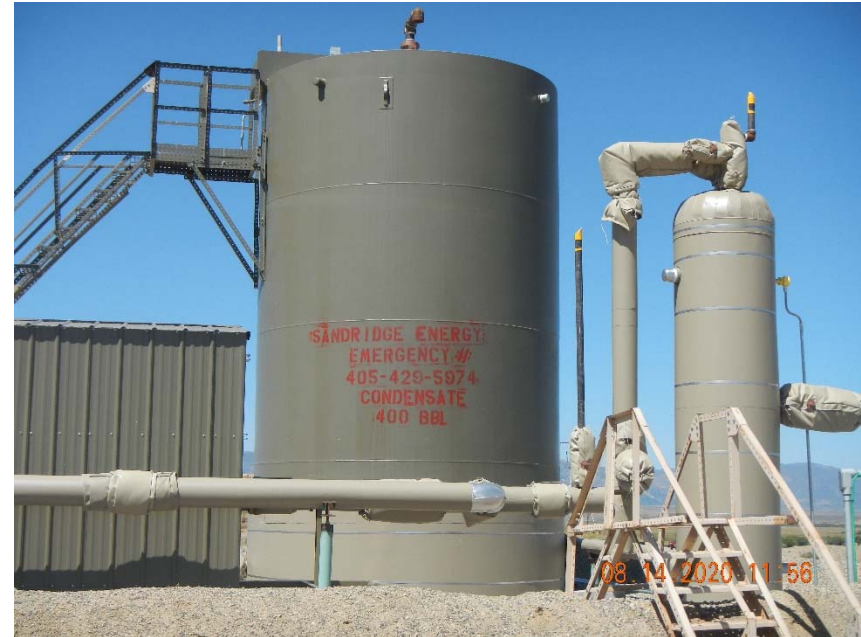
Photo 2. No NFPA diamond on tank label.
