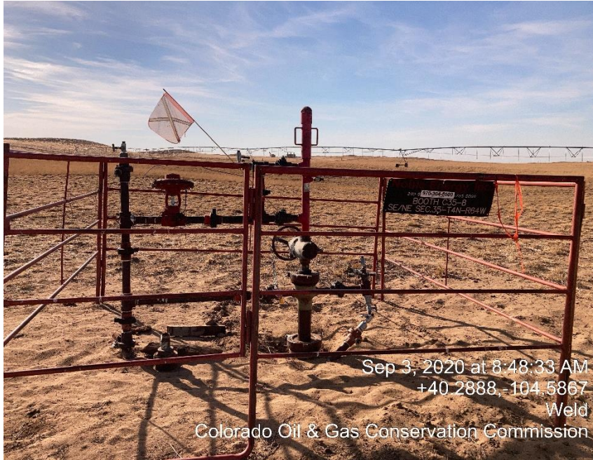
Photo #1 Well & No Leak
