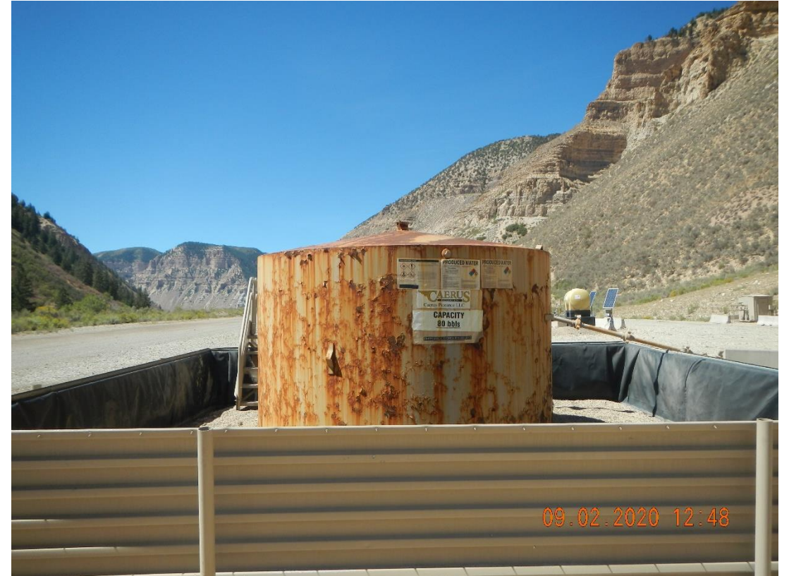
Tank is rusted and peeling paint.
