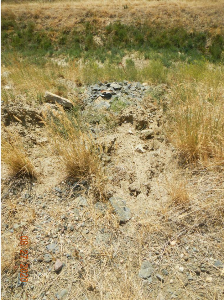
Photo#6: Erosion at pad edge; view down fill slope.
