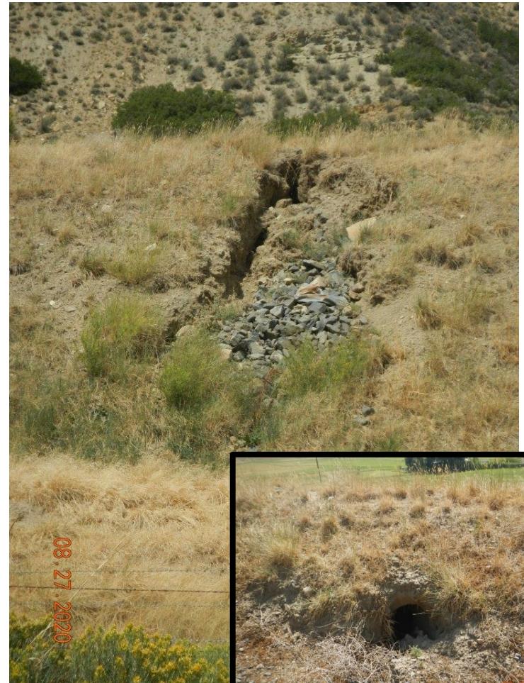
Photo#7: Washout; view from base of fill. Insert of top of slope and believed tunnel/wormhole origination.
