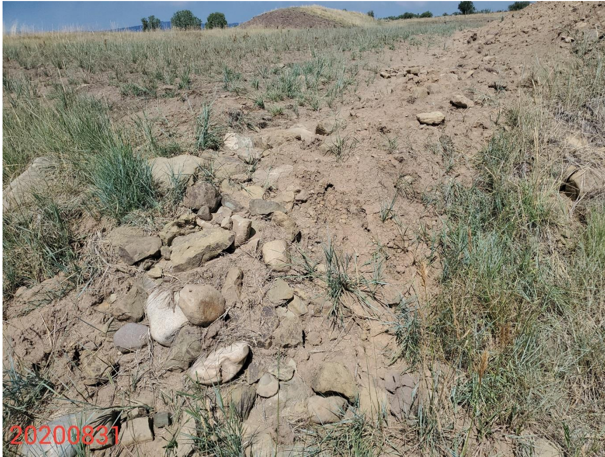
Photo 2: Photo taken from the outlet of the western stormwater ditch. Photo shows outlet/ditch has not been constructed in accordance with good engineering practices; Outlet remains insufficient to stabilize slopes and allow sediment laden-free stormwater discharge.
