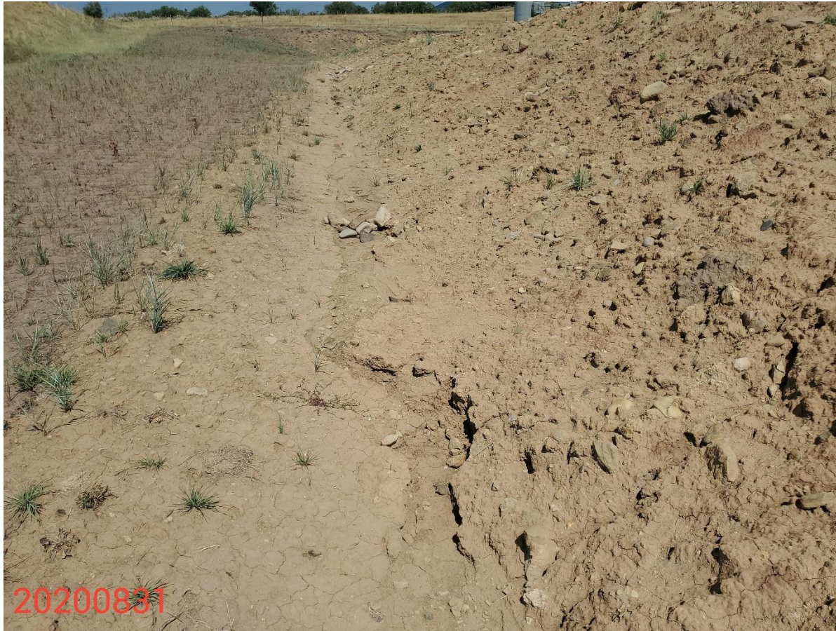
Photo 5: Photo taken from the western stormwater ditch. Photo shows Channel incision/erosion evident. Operator has implemented rock checks/velocity check within ditch. BMP appears insufficient and has not been installed in accordance with good engineering practices.
