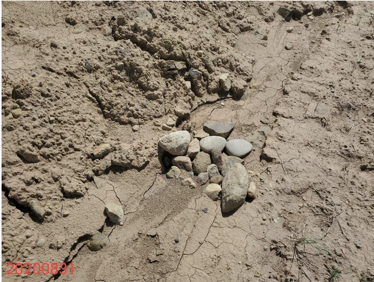
Photo 6: Photo of rock check/velocity check within ditch. See comments under photo 5.
