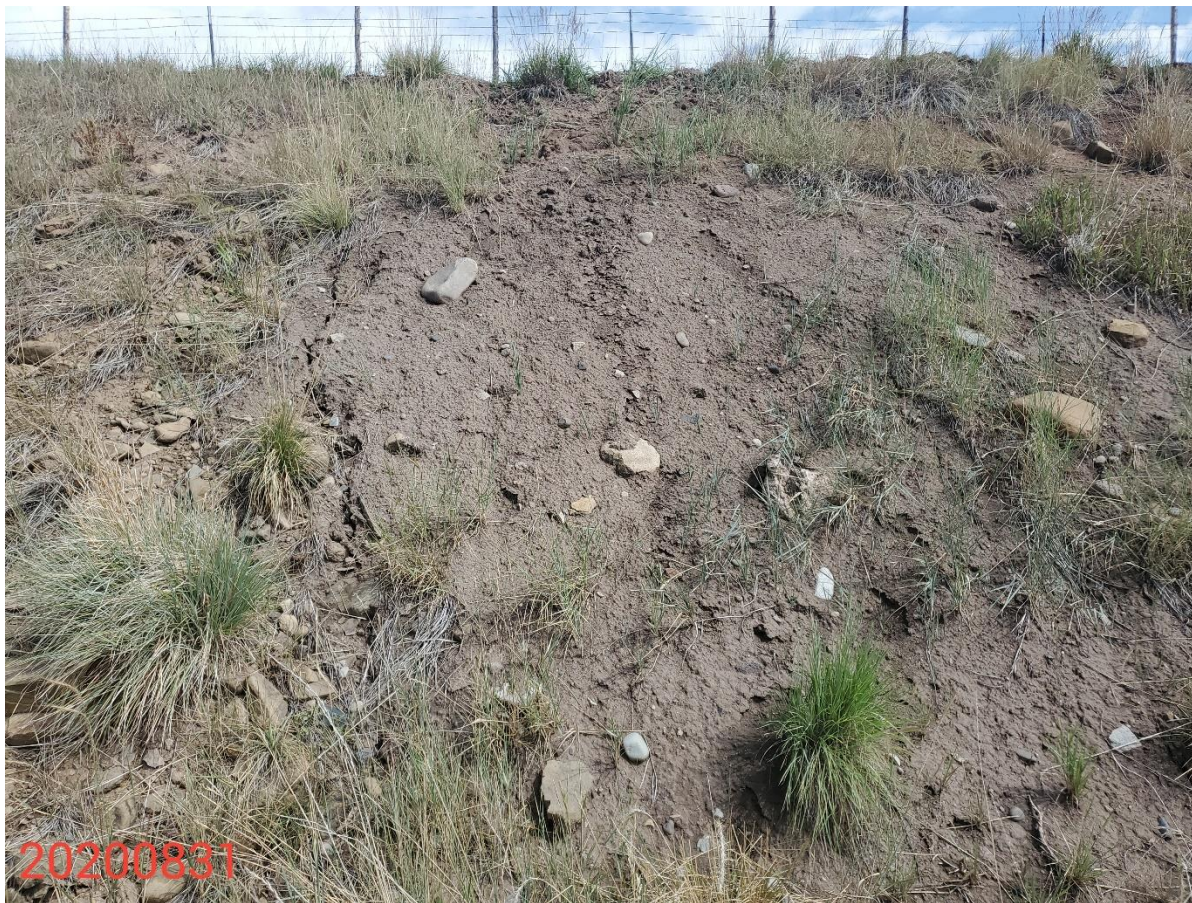
Photo 5: Photo taken from the cut slope on the north end of the Location. Photo shows BMPs to protect and stabilize the slopes remain missing or insufficient. Erosion degradation is recurring.
