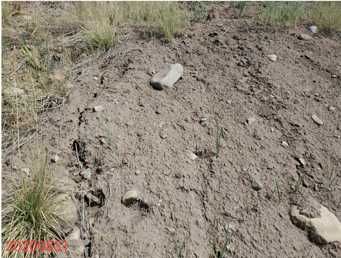
Photo 6: Photo taken from the cut slope on the north end of the Location. Photo shows BMPs to protect and stabilize the slopes remain missing or insufficient. Erosion degradation is recurring.
