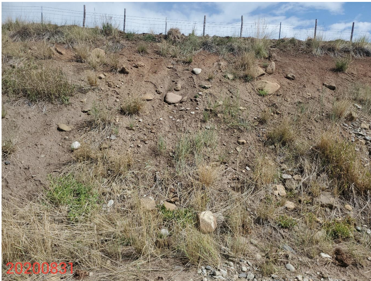
Photo 4: Photo taken from the cut slope on the north end of the Location. Photo shows BMPs to protect and stabilize the slopes remain missing or insufficient.
