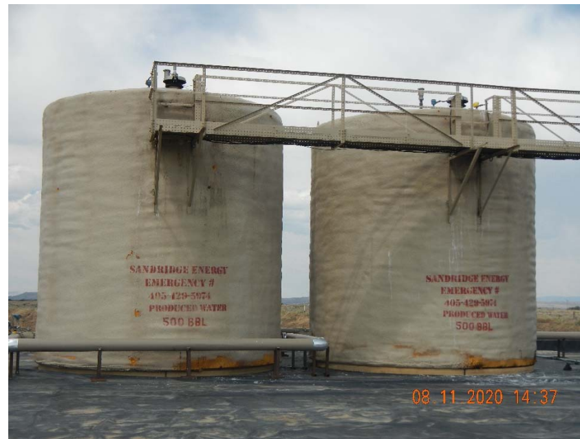
Photo 2. No NFPA diamond on tanks.
