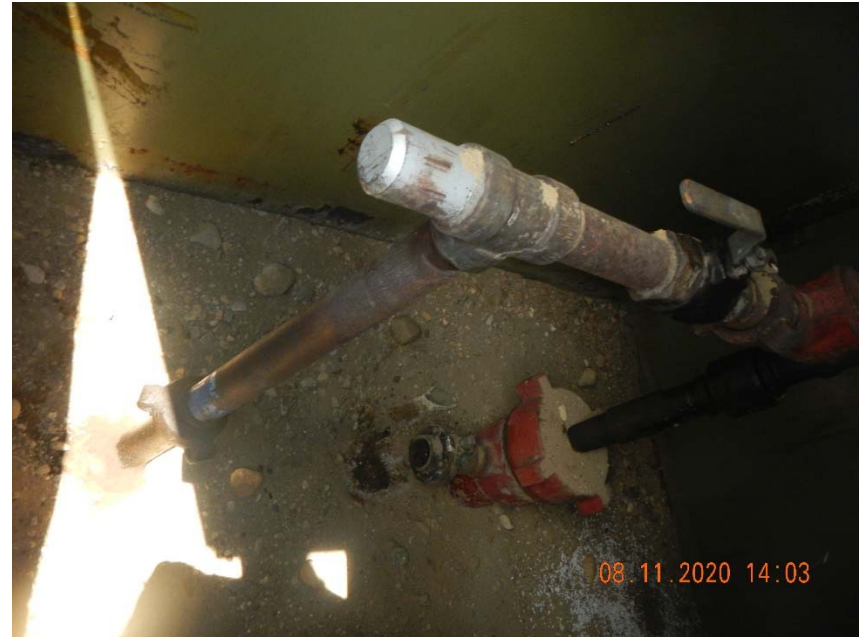
Photo 2. Photo of wellhead inside housing.
