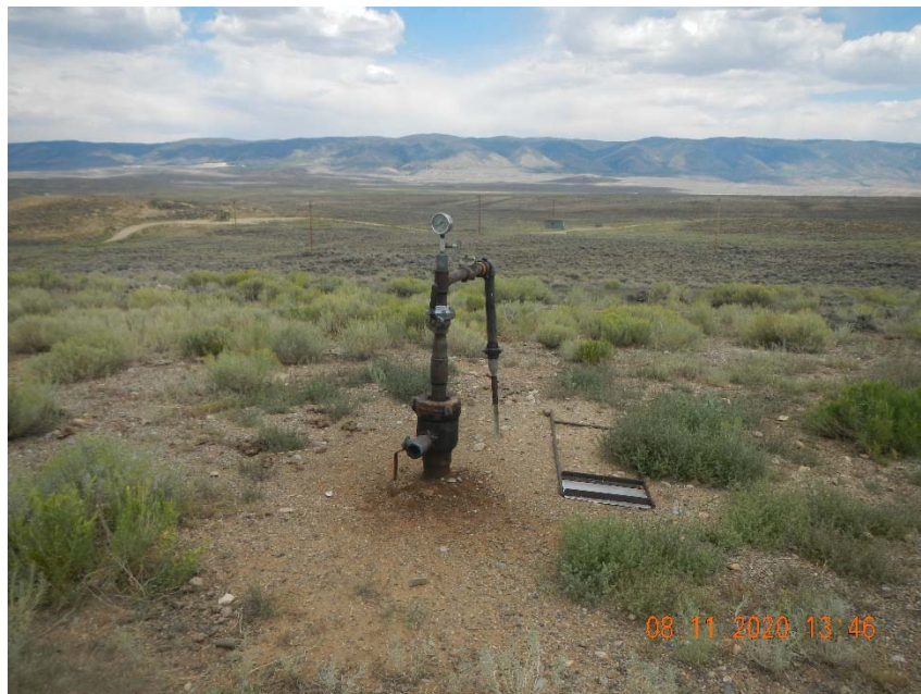
Photo 1. Overview of location taken facing east. Stained soil at wellhead. Wellhead sign knocked over.
