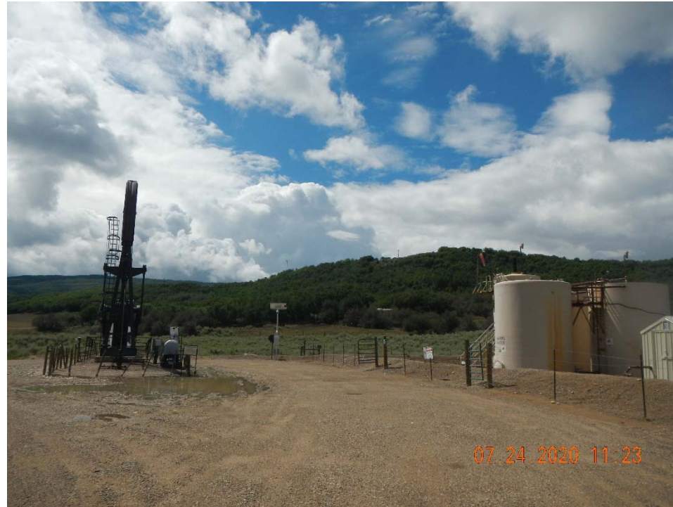
Photo 1. Overview of location taken facing south.
