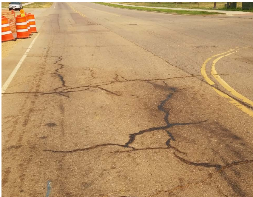
Oil-stained pavement where liquid hydrocarbons surfaced in westbound lane of Tipple Parkway
