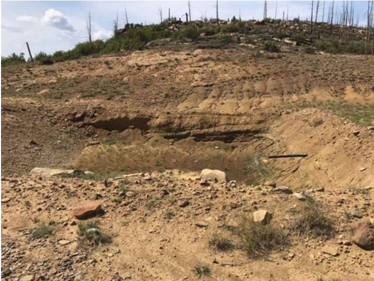
PHOTO 1: THE REMAINING PIECES OF PIT LINER MATERIAL HAVE BEEN REMOVE FROM THE PRODUCTION PIT.
