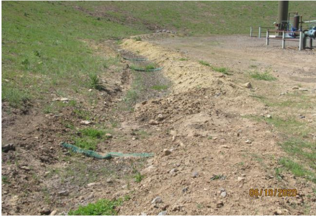
Berm Material within the Dewatering Channel on the Gunderson 20-03 Pad
