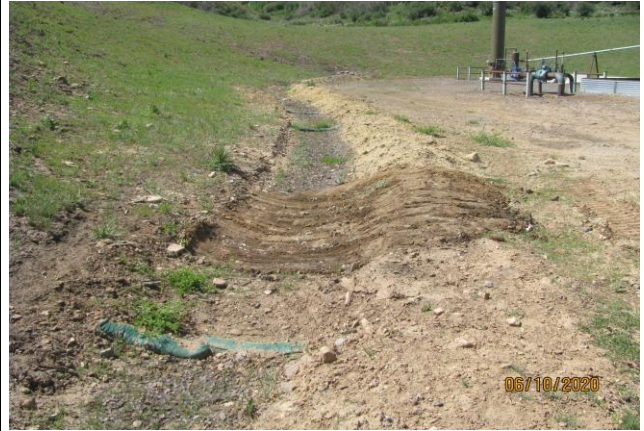
Berm Repaired on the Gunderson 20-03 Pad
