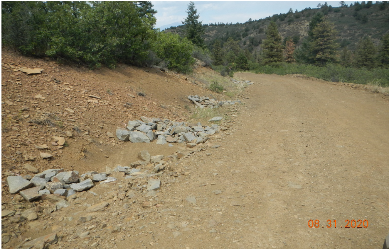
Photo 3. There are rock check dams installed along the road.
