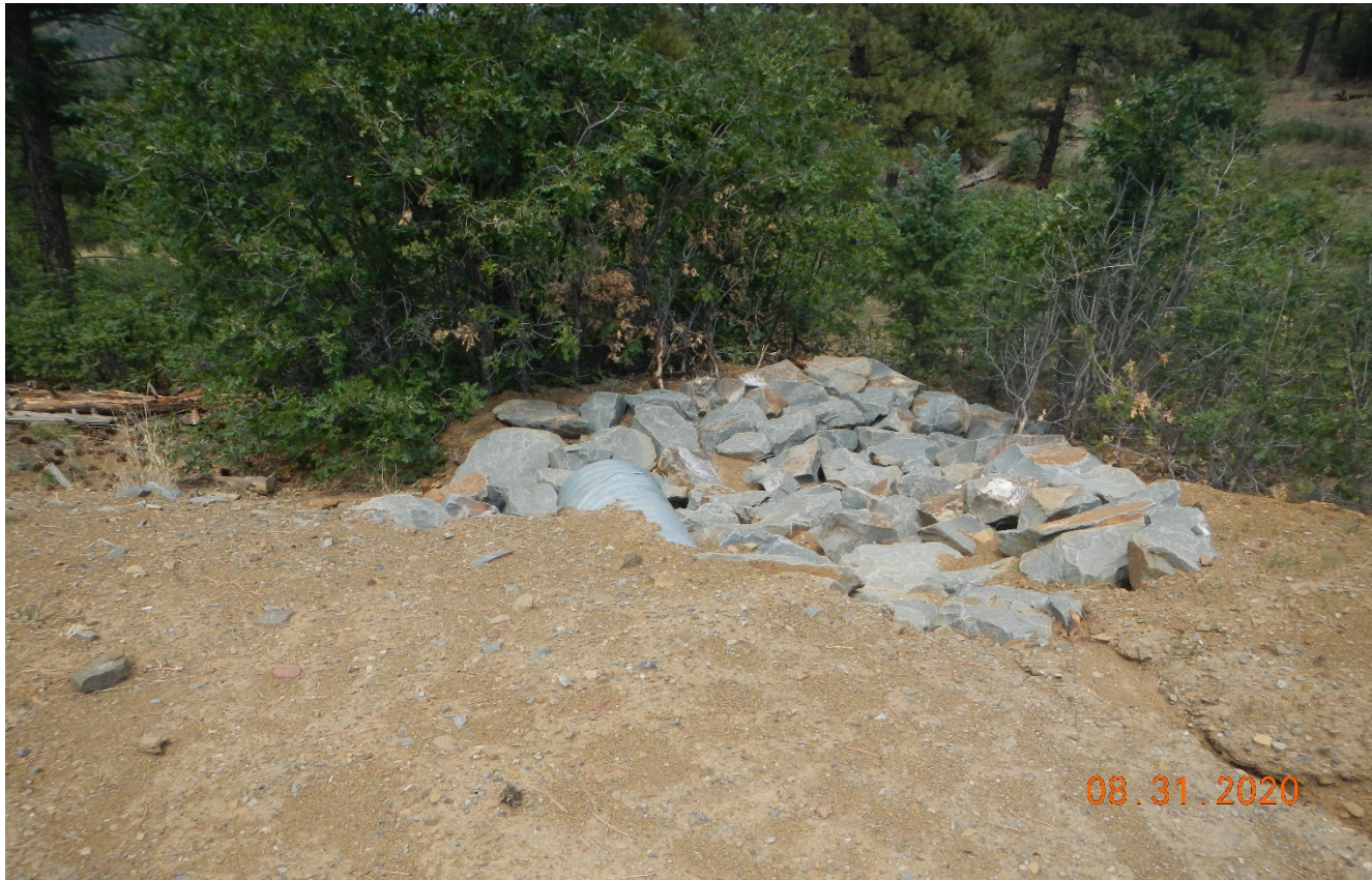
Photo 2. Outlet protection is installed at the culvert.
