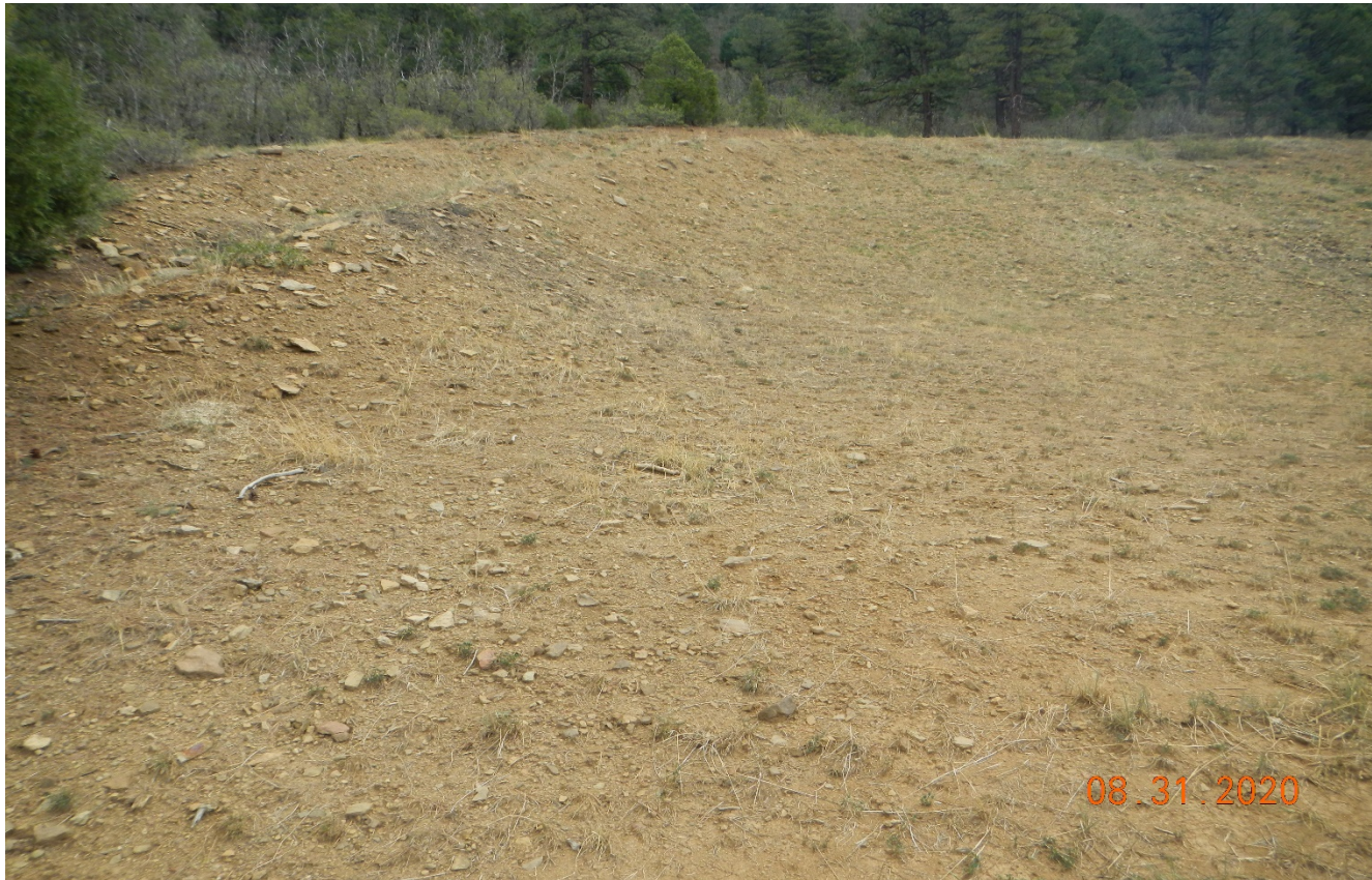
Photo 10. Facing east toward the cut slope. The vegetation has not adequately established along the cut slope.
