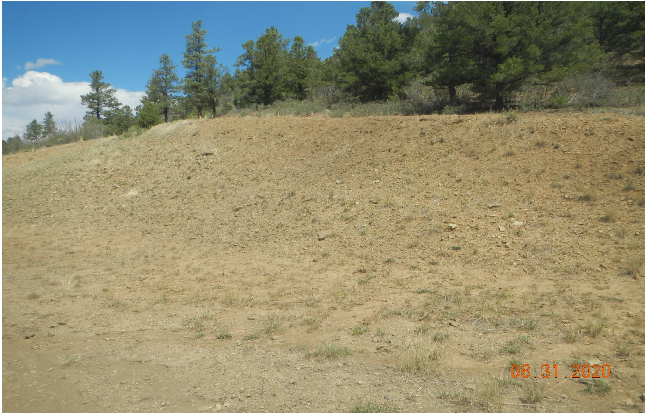
Photo 6. Facing toward the cut slope. The vegetation has not adequately established along the cut slope.
