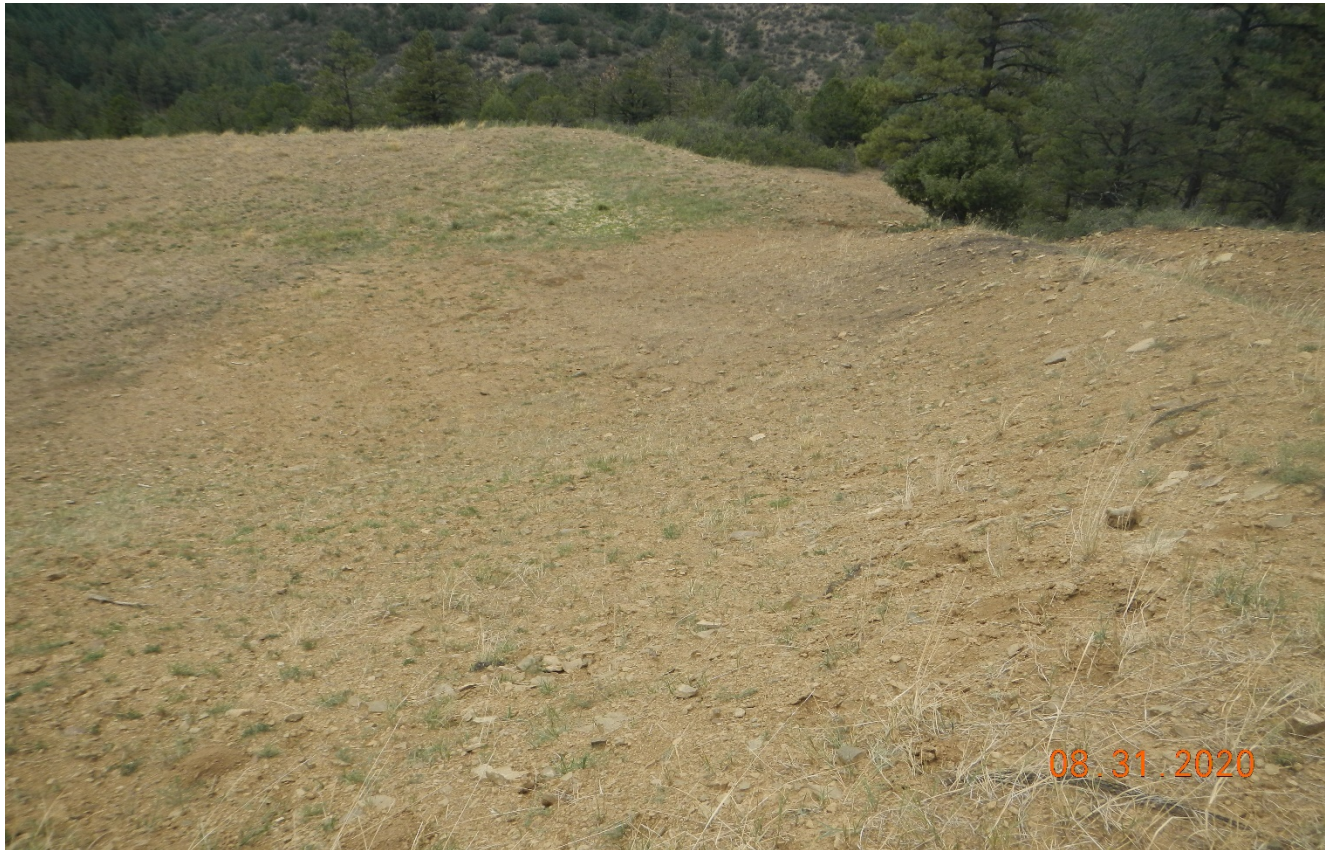
Photo 8. Facing west standing at the top of the cut slope. The vegetation has not adequately established along the cut slope.
