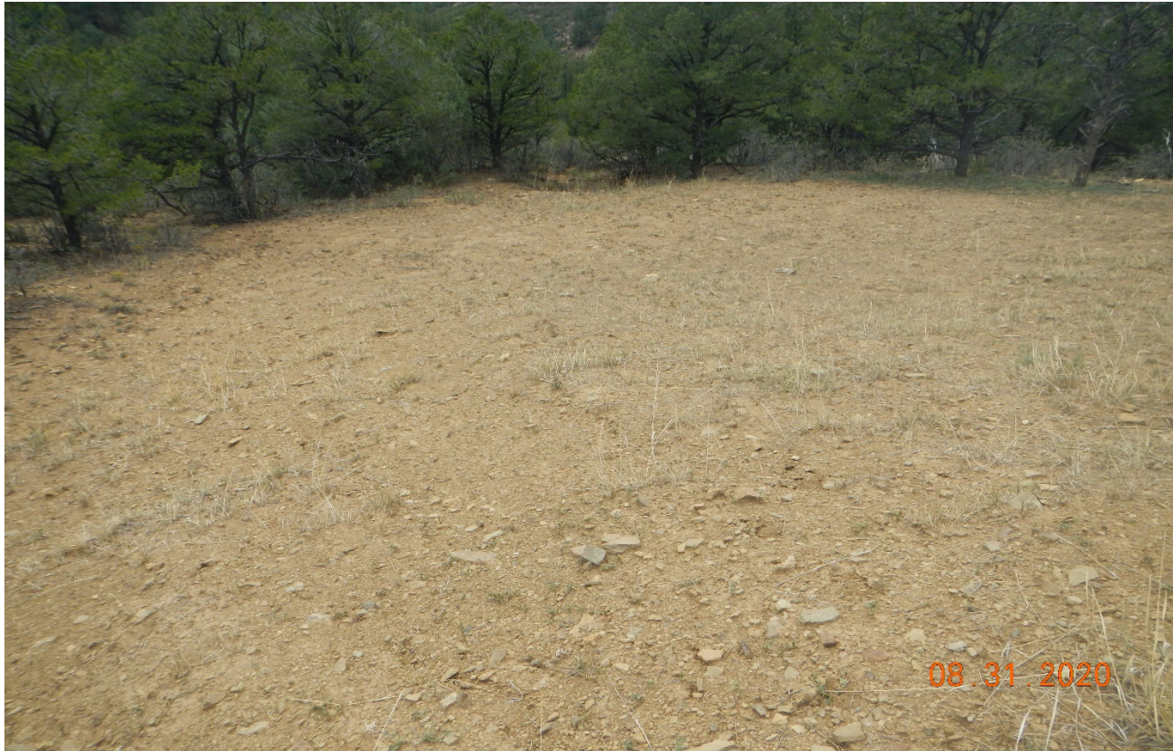
Photo 12. Facing west of the fill slope. The vegetation has not adequately established along the fill slope.
