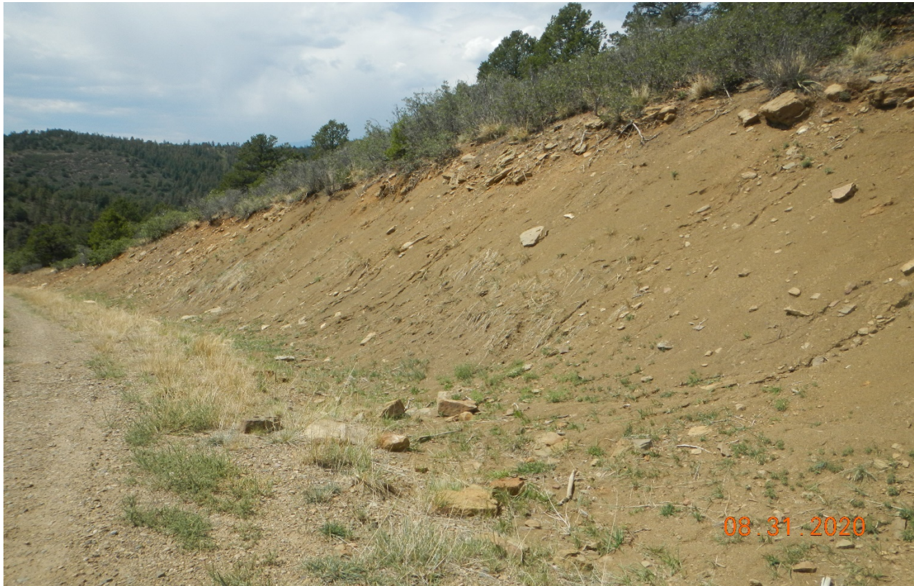
Photo 3. There are areas along the cut slope that are not stabilized.
