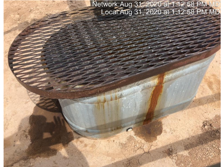
Photo #1817 Containment by pig station full of oily fluids.
