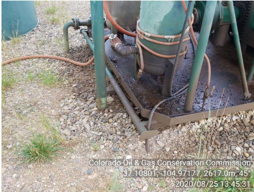
PHOTO 5: AREA OF IMPACTED SOIL AROUND COMPRESSOR.
