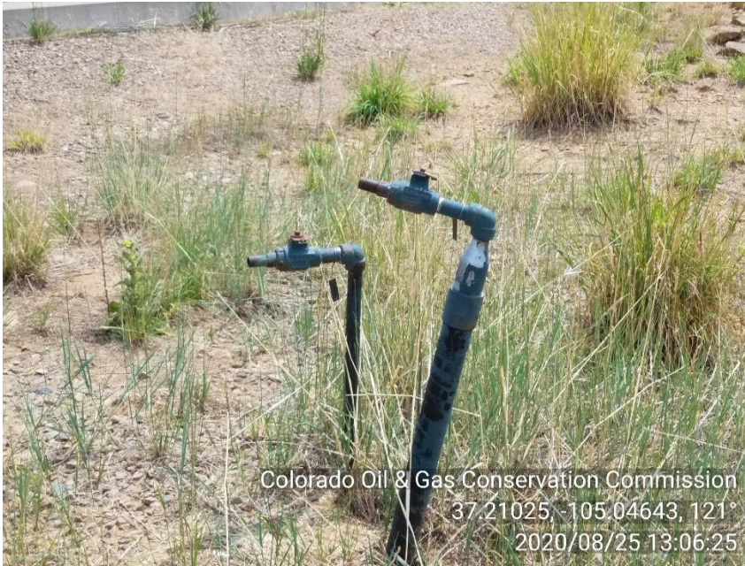
PHOTO 3: UNMARKED UNUSED RISERS NOT LO/TO. REMOVE OR MARK AND LOCKOUT/TAGOUT RISERS, COMPLY WITH RULE 603.f. CA DATE 11-25-20.
