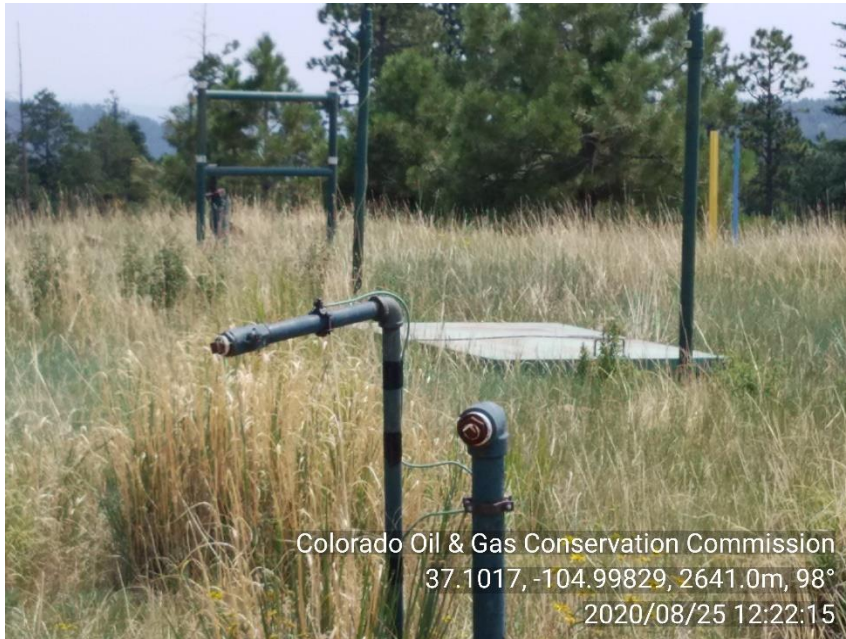
PHOTO 3: UNMARKED UNUSED RISERS ON NORTHWEST EDGE OF LOCATION. REMOVE OR MARK RISERS, COMPLY WITH RULE 603.f. CA DATE 11-26-20.
