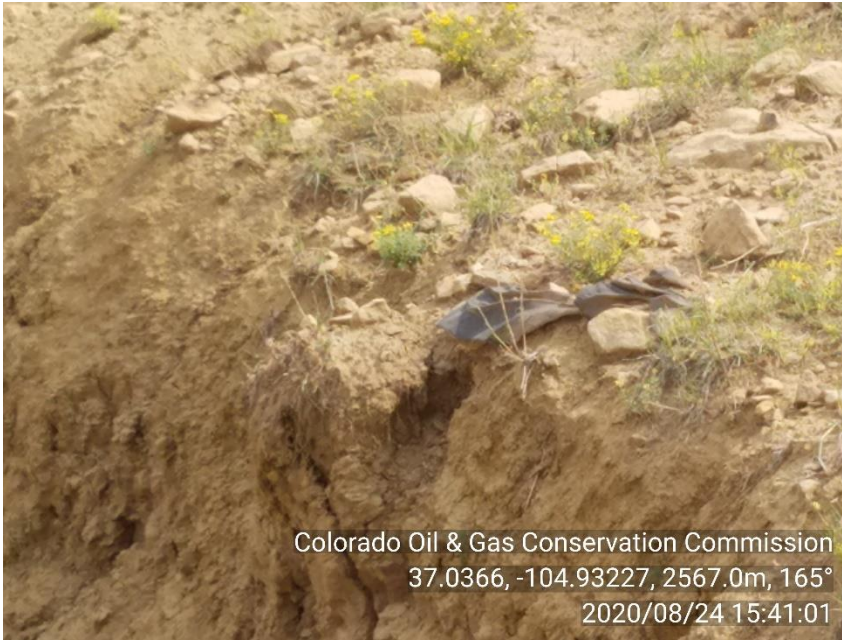
PHOTO 5: MORE IMAGES OF PIT LINER ON TOP EDGE OF PIT. REMOVE ALL TRASH IN AND AROUND PIT, COMPLY WITH RULE 603.f. CA DATE 9-8-20.
