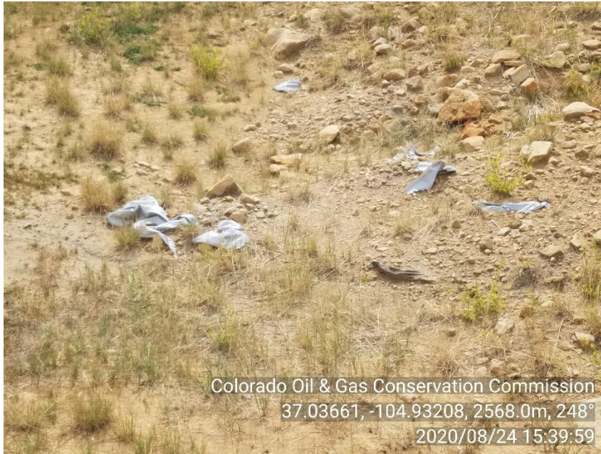
PHOTO 3: TRASH IN EARTH PIT (PIECES OF PIT LINER LEFT IN PIT). REMOVE ALL TRASH IN AND AROUND PIT, COMPLY WITH RULE 603.f. CA DATE 9-8-20.
