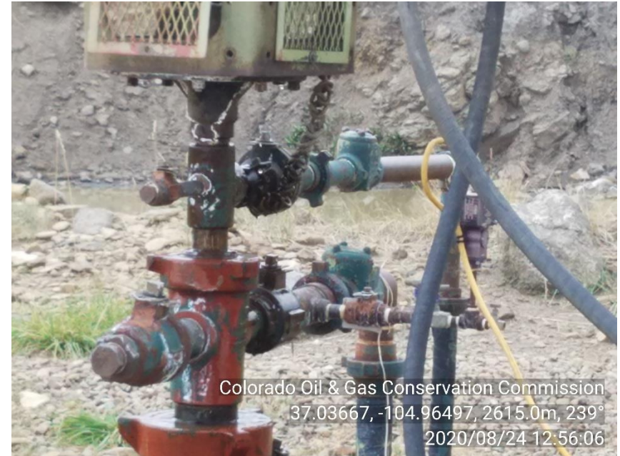
PHOTO 4: CLOSER IMAGE OF PACKING LEAK, FOLLOW GUIDANCE GIVEN ON PHOTO 3.
