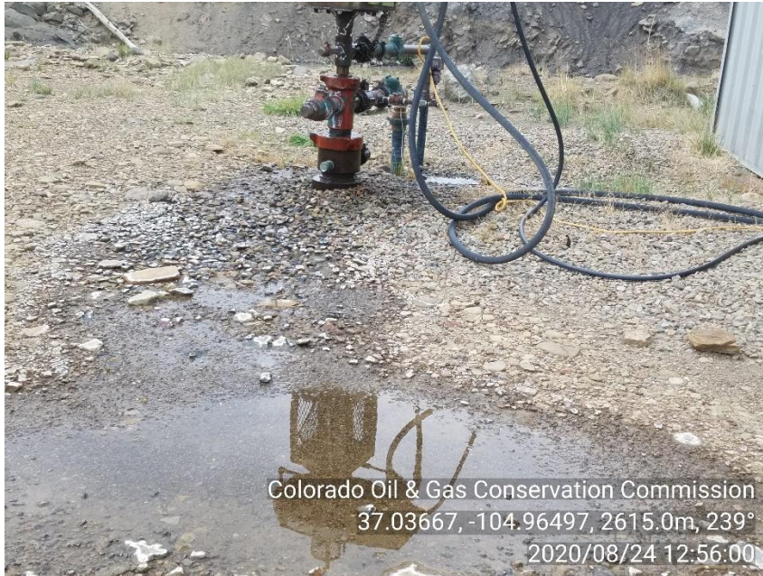
PHOTO 3: TBG PACKING IS LEAKING PRODUCED WATER. REPAIR PACKING (THERE IS LITTLE TO NO STANDING FLUID ON THE GROUND), COMPLY WITH RULE 907.c. AND Securely fasten all valves, pipes, and fittings to ensure good mechanical condition, inspect at regular intervals and maintain in good mechanical condition per Rule 605.d. CA DATE 8-25-20.
