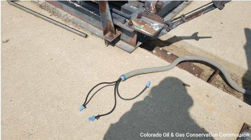
**Photo 5 unused electric wire from electric panel.**
