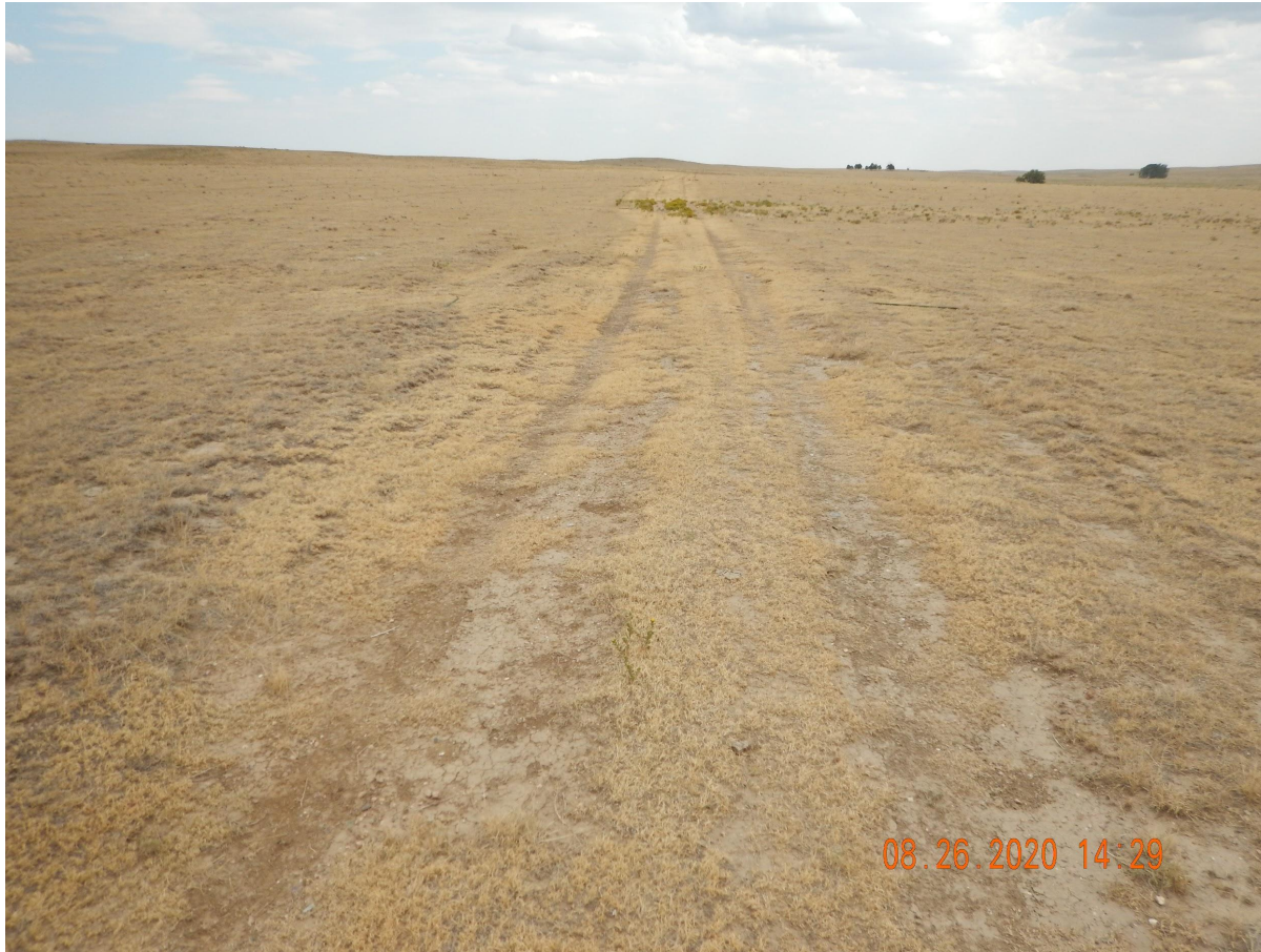
Photo 1. Photo taken from the western access road, facing East. Photo illustrates the access road has not been reclaimed and does not meet Rule 1004 vegetative requirements.
