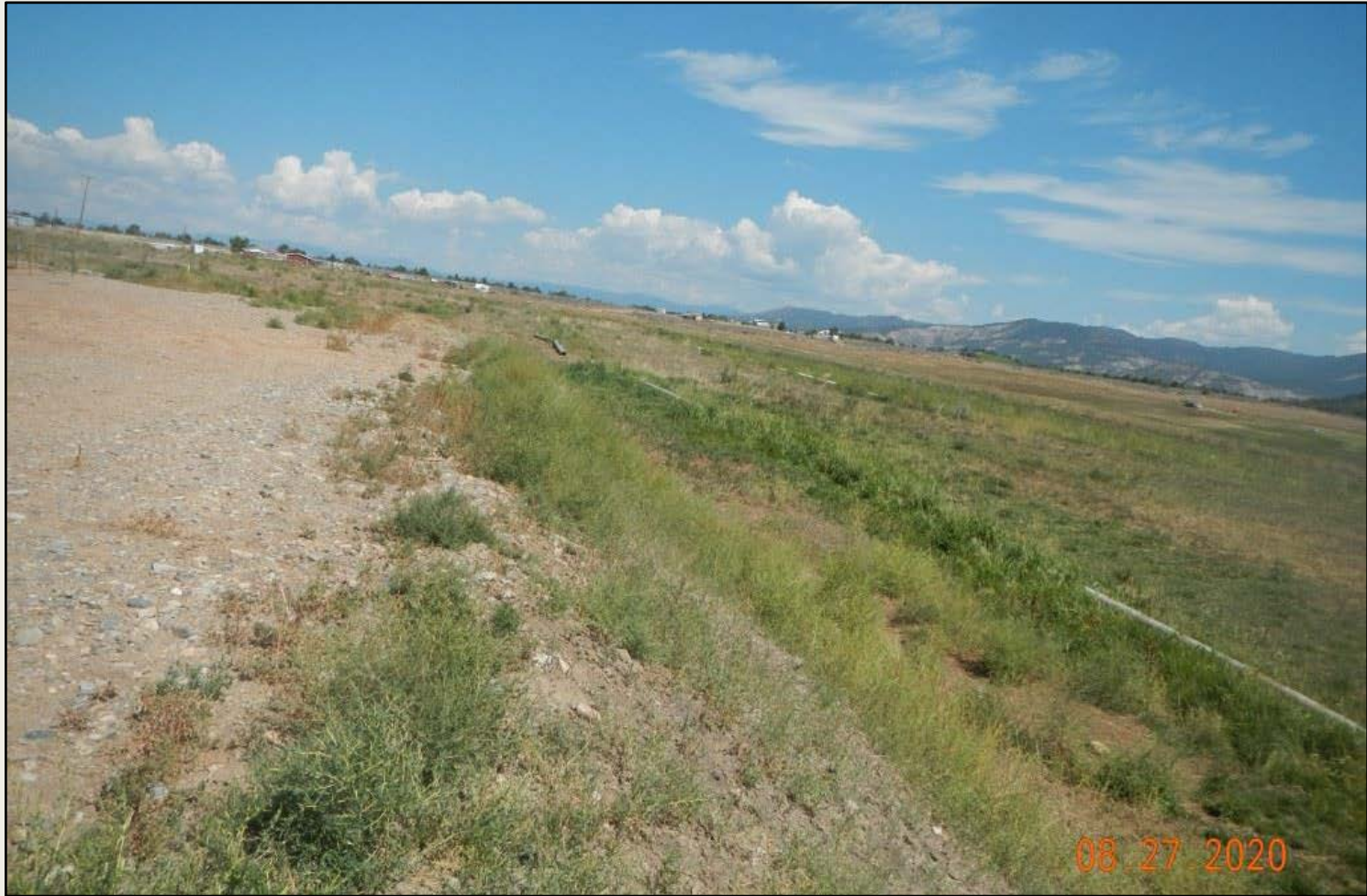
Photo 2. View of the eastern fill slope from the southeastern corner facing northward. Revegetation is progressing outside of irrigation alignment, with western wheatgrass and smooth brome.
