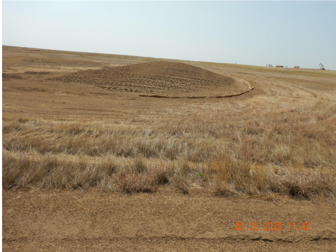
Photo 4. Photo taken from the northwestern location, facing South. Photo illustrates the topsoil stockpile which has been temporarily stabilized with equipment tracking. Wattle BMPs have been installed around the outer perimeter of the stockpile.
