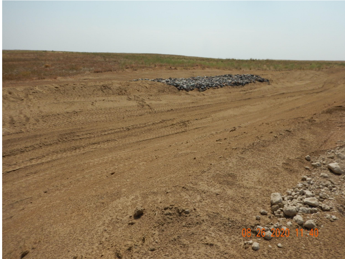
Photo 2. Photo taken from the northeastern location, facing Southeast. Photo illustrates stormwater BMPs- retention area, and a stabilized outlet. Stormwater BMP areas will likely need to be stabilized due to the sandy soil.
