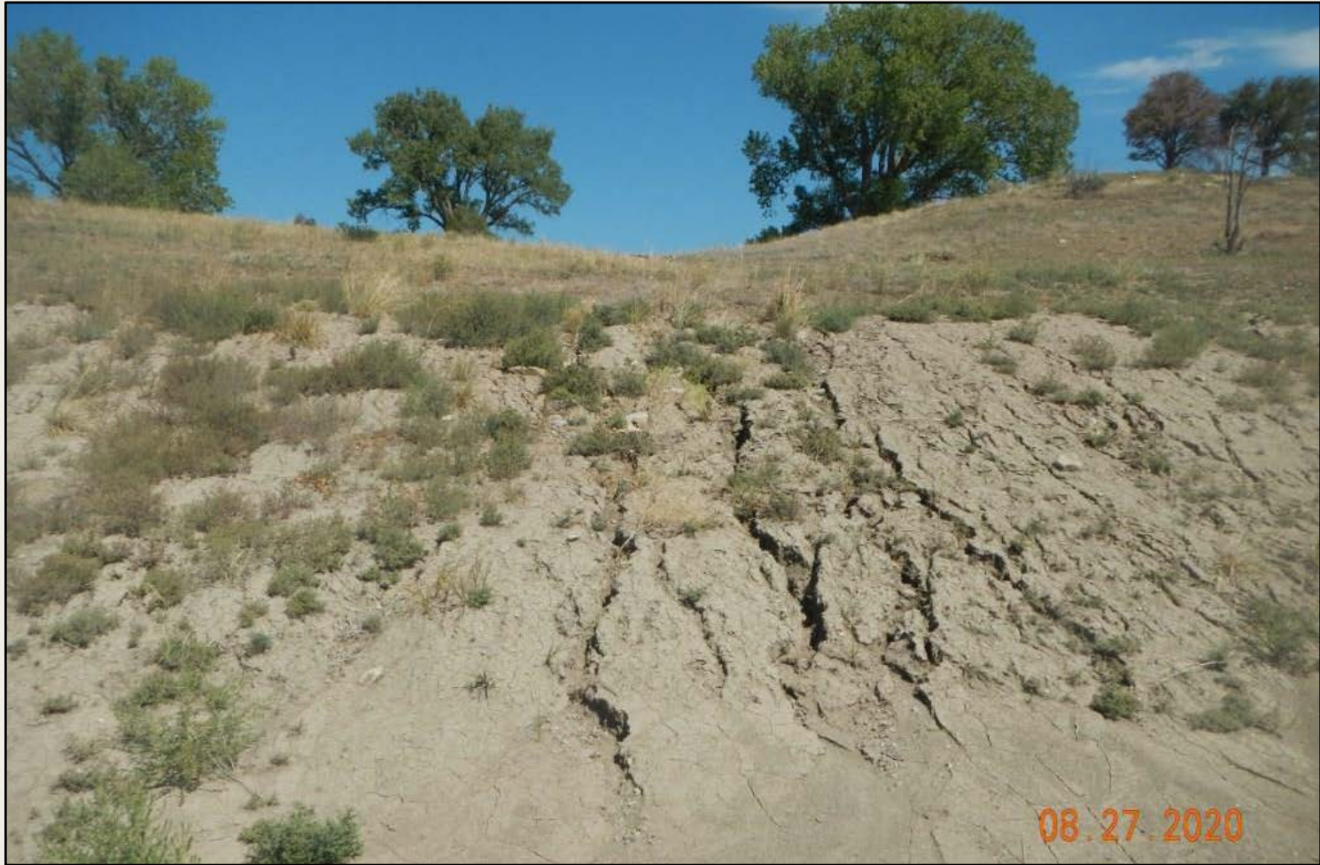
Photo 5. View of erosional rilling and sediment deposition that continues on the well pad cut-slopes.
