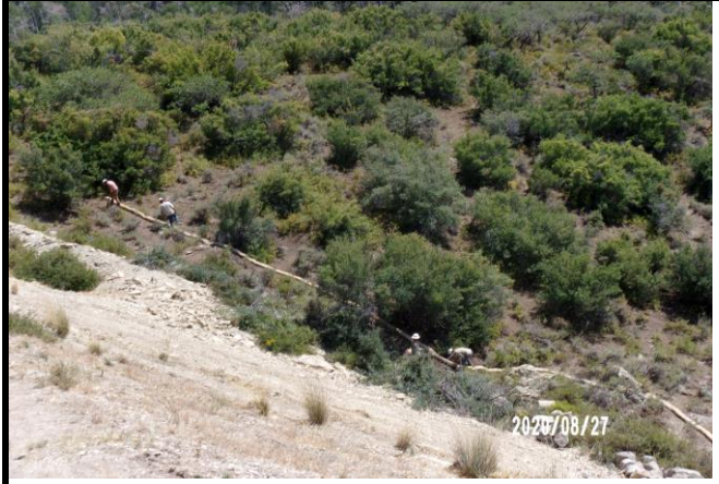
Wattle Installation on the C.C. 697-15-01 Pad
