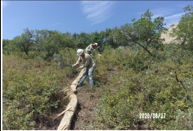
Wattle Installation on the C.C. 697-15-01 Pad
