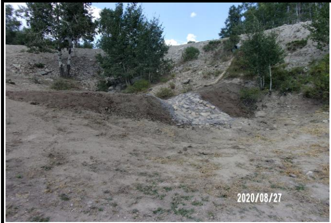
Sediment Trap Installation below the Culvert Outlets
