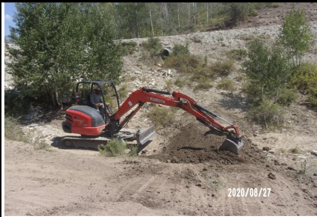
Sediment Trap Installation below the Culvert Outlets
