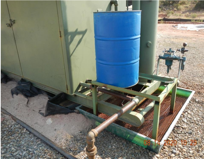
55 gal. drum on secondary containment.
