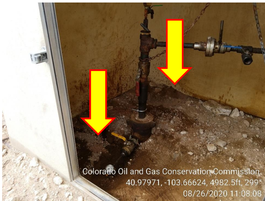
Photo 1 – Wellhead, Stained Soil
