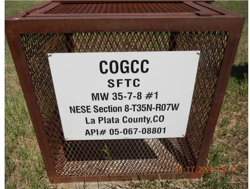
Monitor Well 35-7-8 #1 location sign and protective metal cage.
