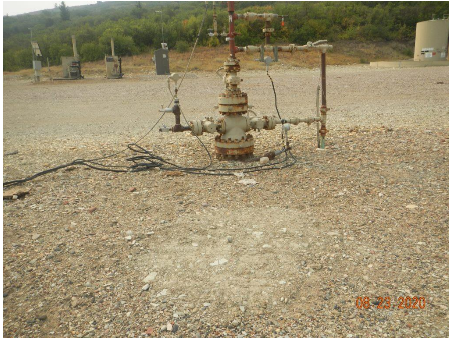
Photo#2: Subsidence repaired.
