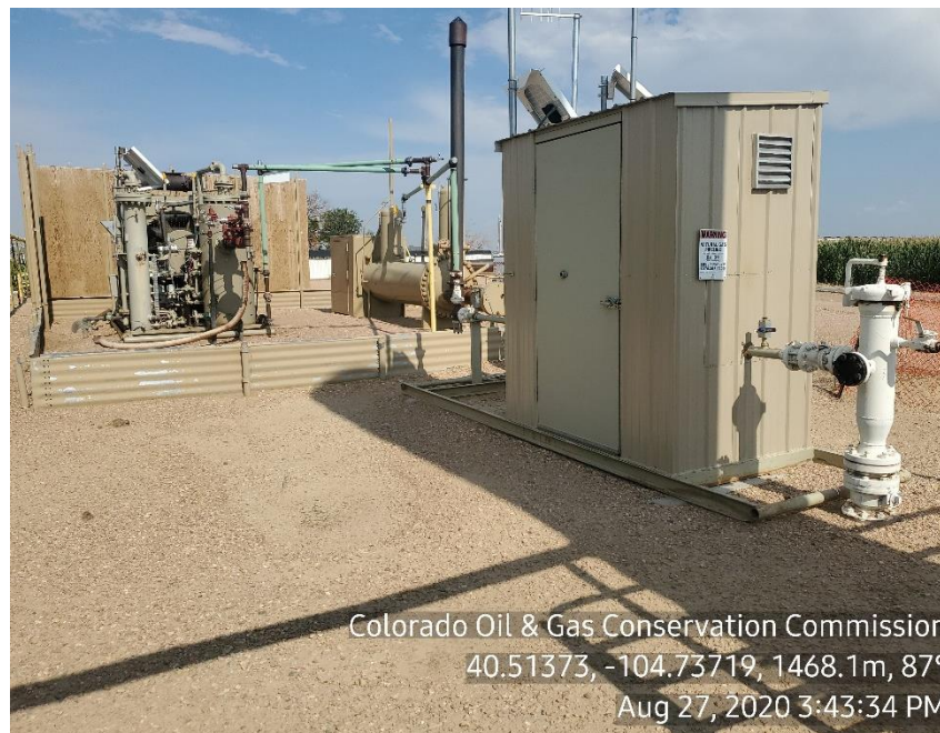
Photo 3: Unused gas meter removed
