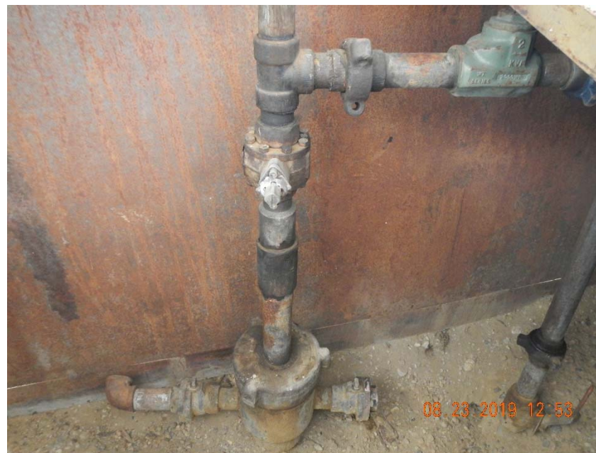
Photo 2. Photo of wellhead inside housing.
