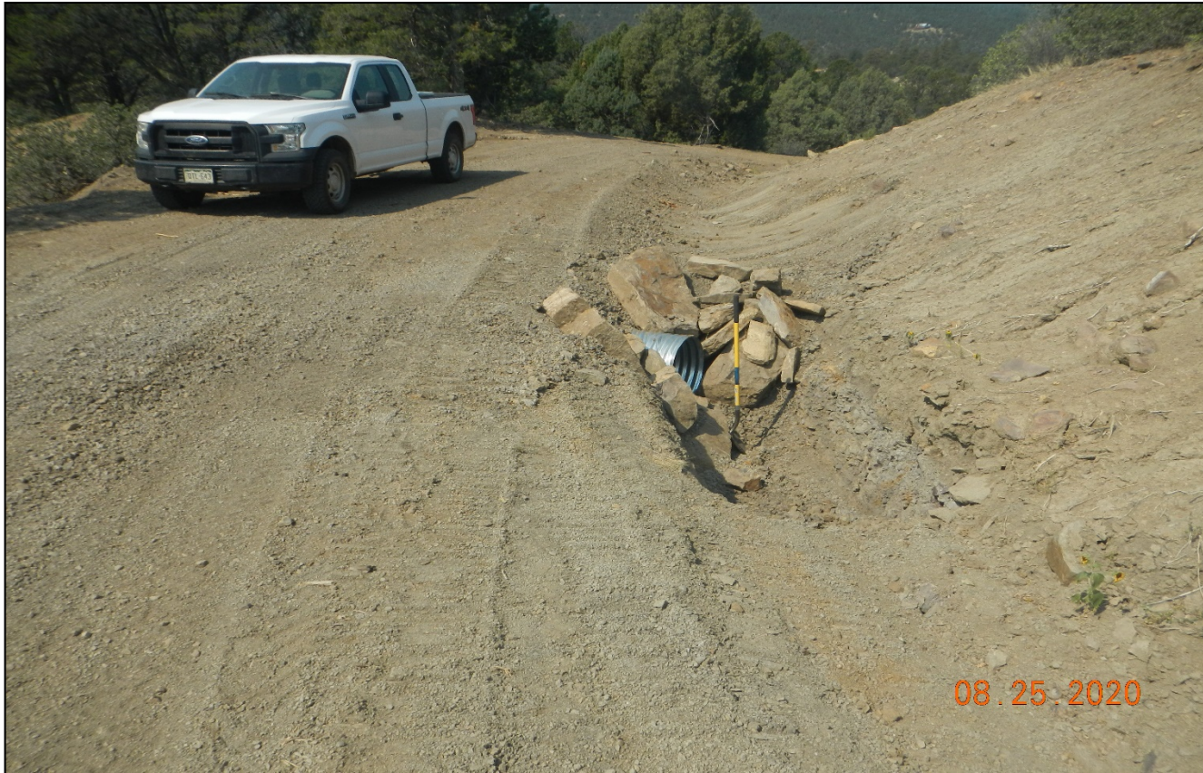
Photo 8. Facing toward the culvert inlet installed along the road.
