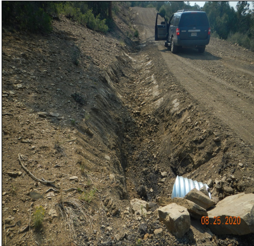
Photo 4. There are culverts installed along the road ascending this hillside.
