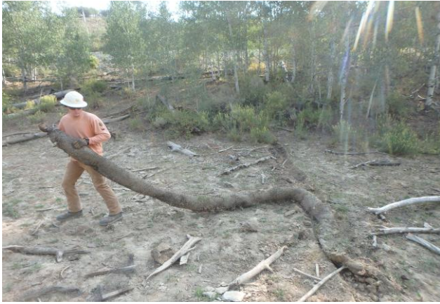
Removing Wattle from the Lower Loop Road
