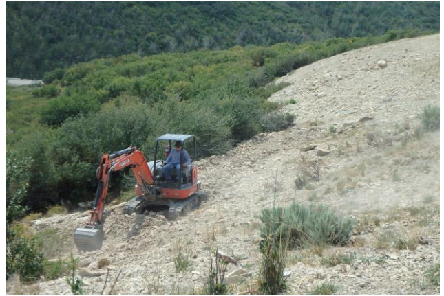
Preparing the CC 697-16-16 for Wattle Installation
