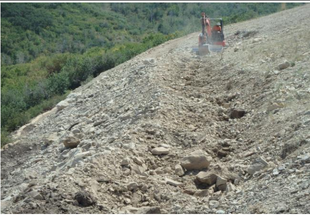
Pockmarking Previously Installed Water Bars
