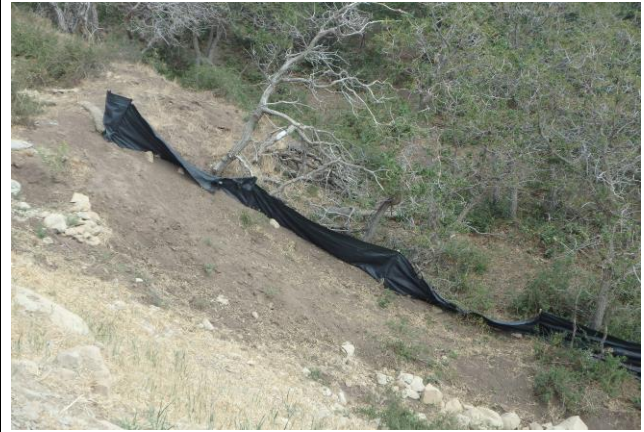
Damaged Silt Fence on CC 610-21-41
