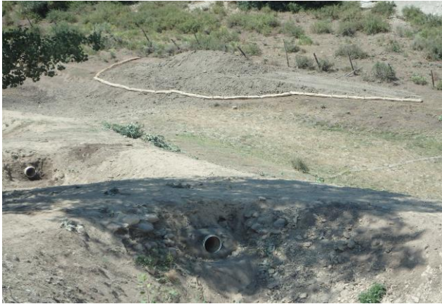
BMPs Installed Below the Lower Loop Road
