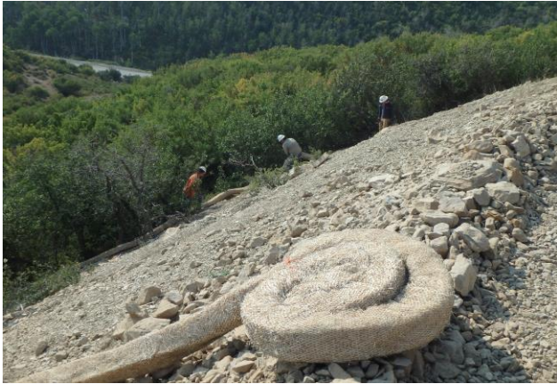
Installing Excelsior Wattle on CC 697-16-16 Pad
