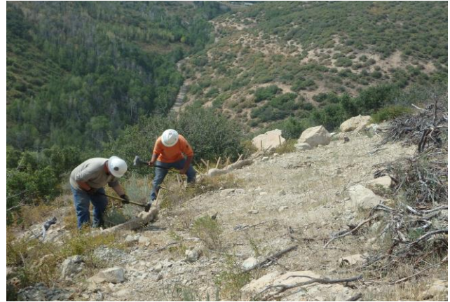
Installing Excelsior Wattle on CC 697-16-16 Pad
