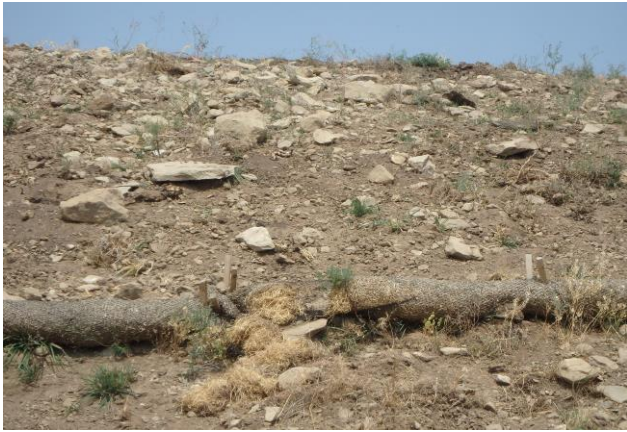
Wattle Damaged on the CC 610-24-43
