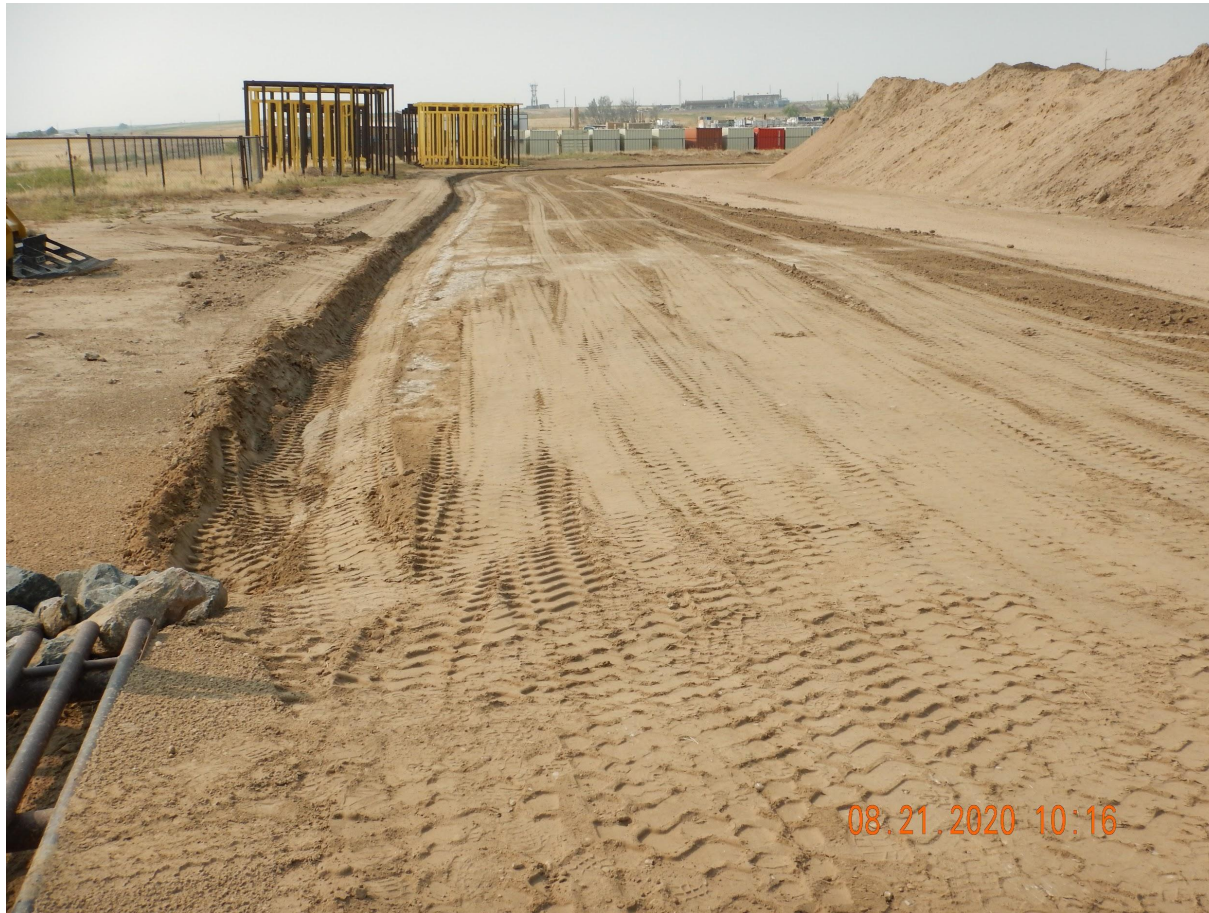
Photo 3. Photo taken from the gated entrance, facing South. Photo illustrates stormwater controls have been installed to manage stormwater that flows onto and off the location.
