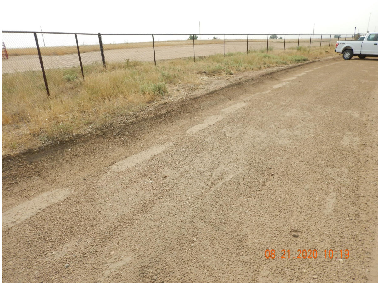
Photo 4. Photo taken from the northeastern location, facing South. Photo illustrates stormwater controls have been installed to manage stormwater that flows onto and off the location.
