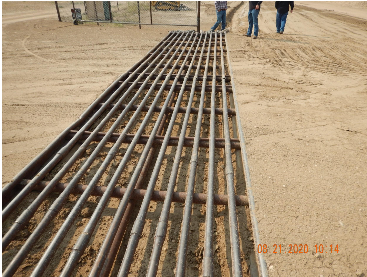
Photo 2. Photo taken from the gated entrance, facing South. Photo illustrates stormwater controls have been installed to manage stormwater that flows onto and off the location.
