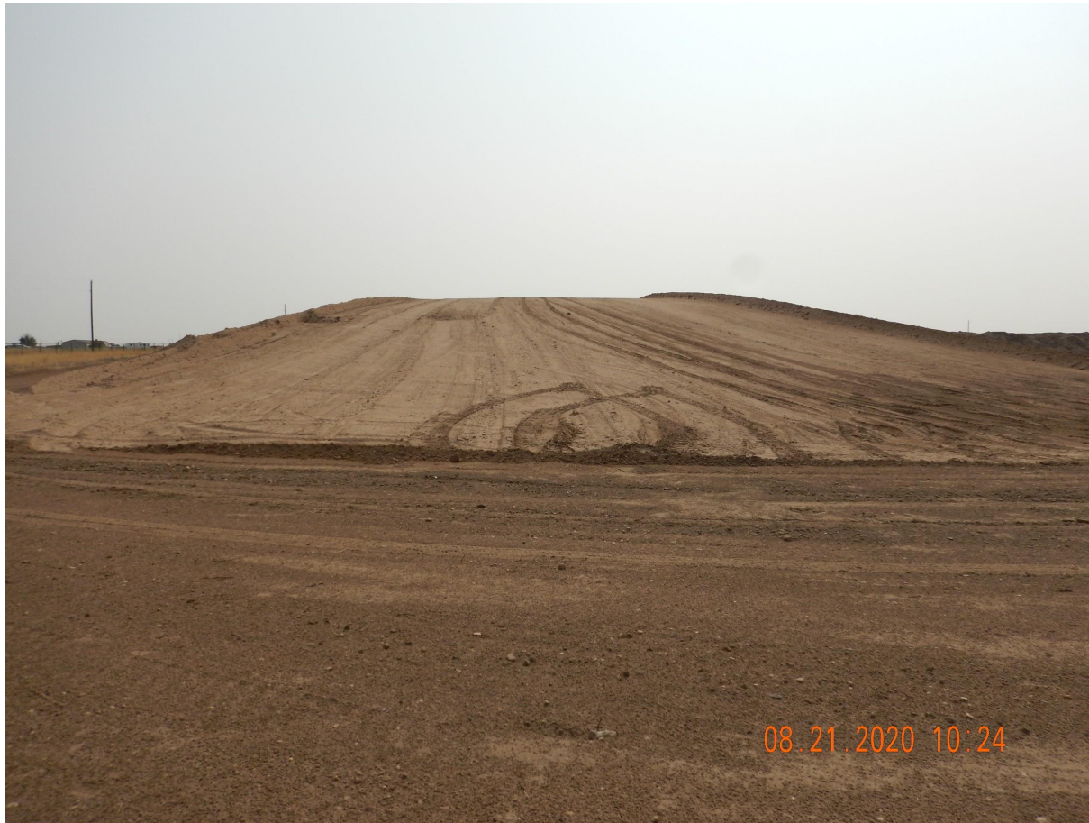
Photo 6. Photo taken from the northwestern location, facing East. Photo illustrates a stockpile of fill material used for interim reclamation locations.
