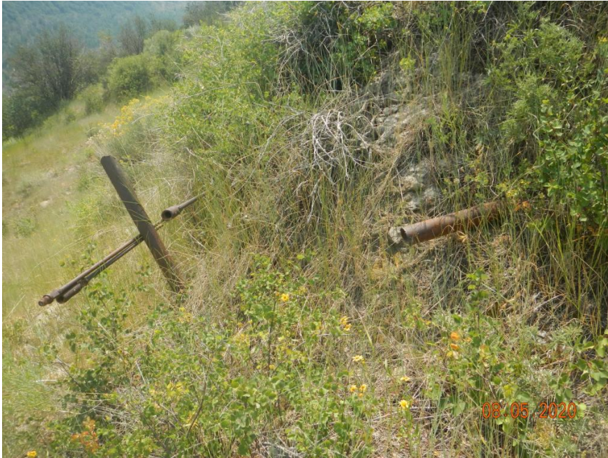
Photo#7: Pipes/lines/riser daylighting from bank below pad.
