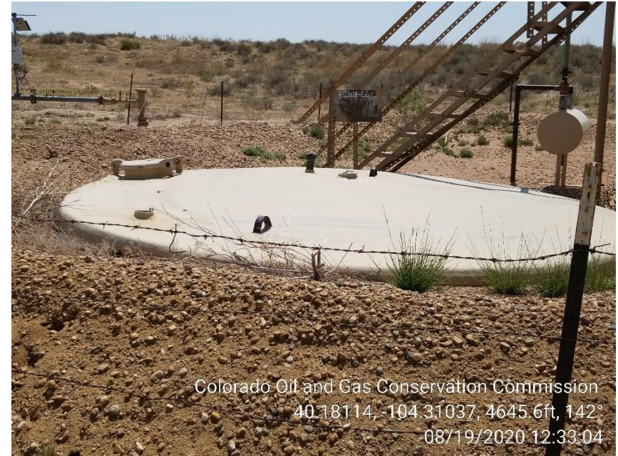
Photo 6 – Produced Water Tank missing Content, Capacity and NFPA Labels
