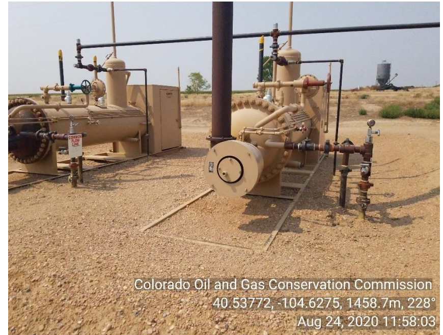
Photo 4: Risers removed
