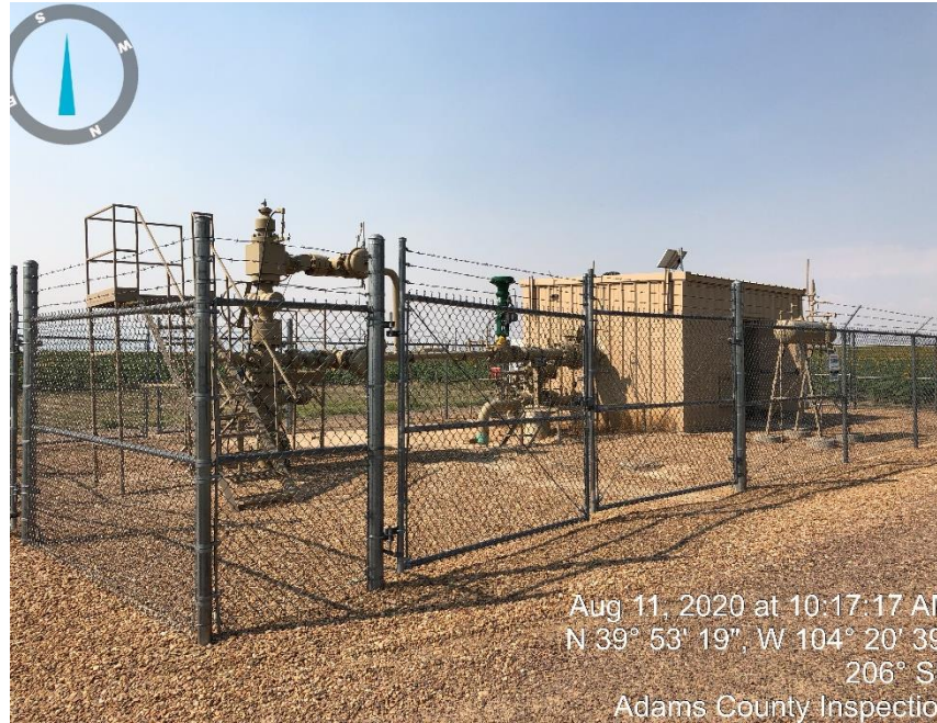
Photo #1 Well head & separator house.
