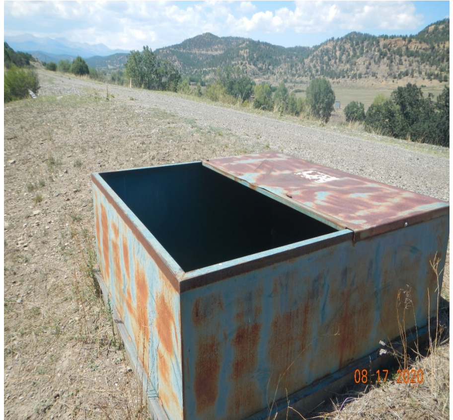
Photo 1. There is a metal pipeline box near the location which the lid has blow off. This needs to be repaired to prevent wildlife entry.
