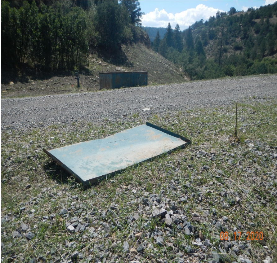
Photo 1. There is a metal pipeline box near the location which the lid has blow off. This needs to be repaired to prevent wildlife entry.
