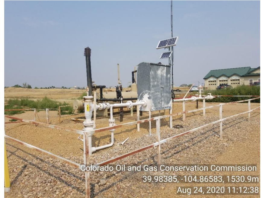
Photo 2 meter run and separator
