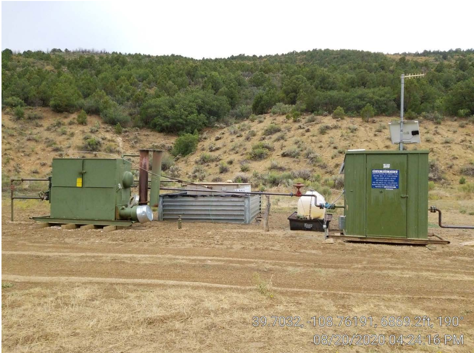
Photo 2. Separator, tank, meter building.
