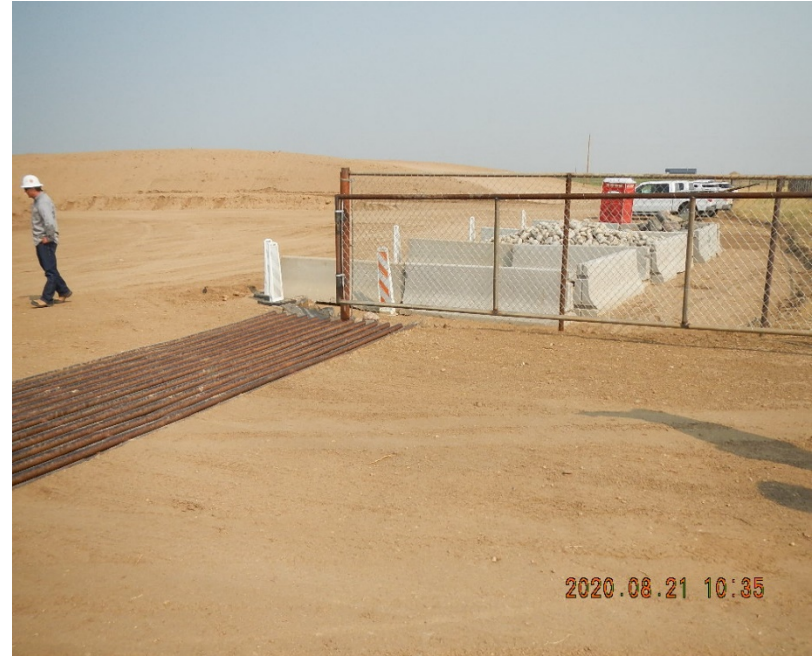
Entrance to CE&P Facility. Note: Gate is now secured and storm water runoff controls have been implemented.
